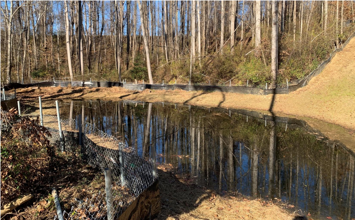
November 29, 2025 Mud excavated from the northern end of pond
