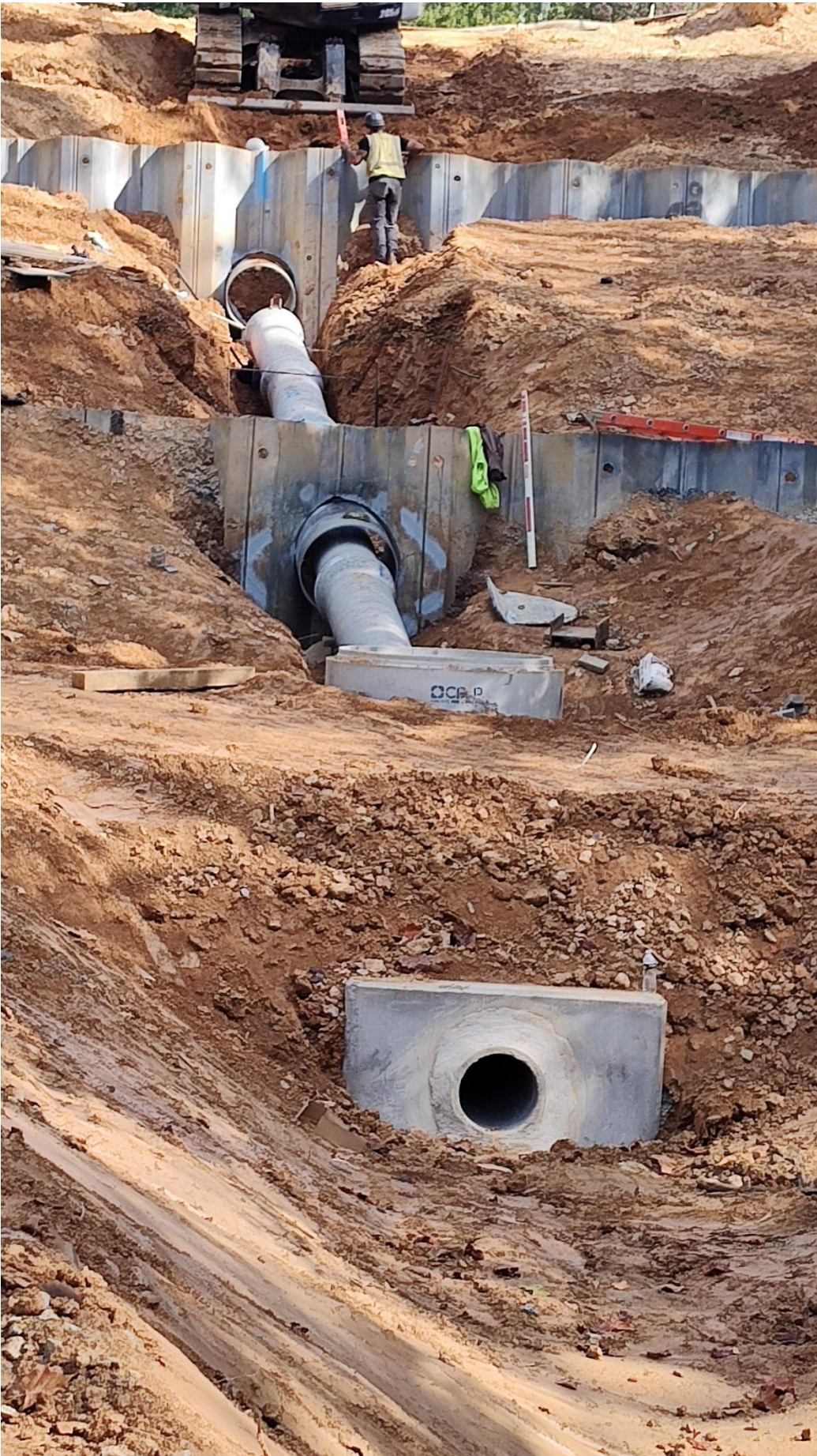
October 10, 2025 Laying the new pipe Vertical steel sheets stabilize the slope
