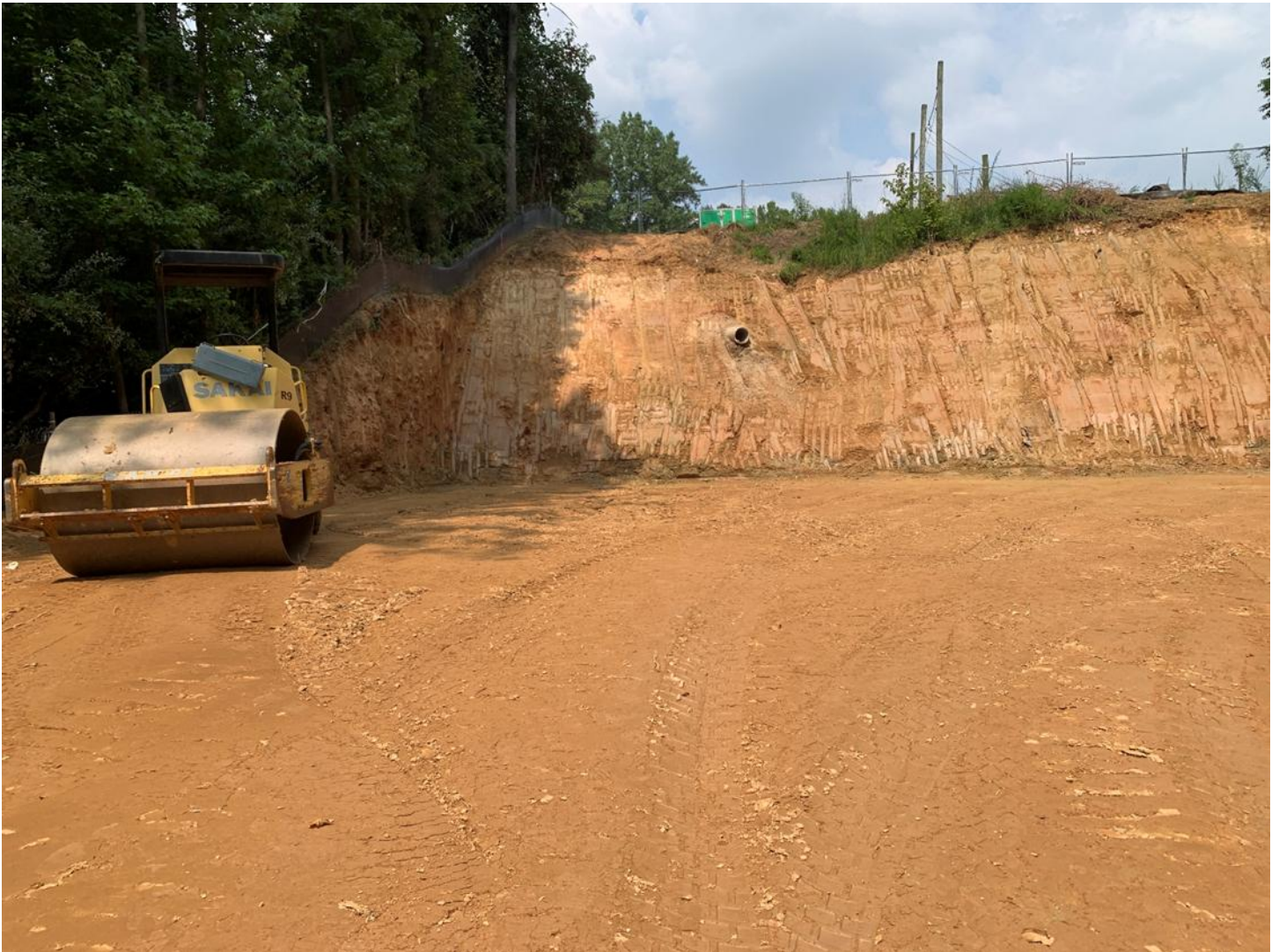
August 7, 2025 Excavating the slope
