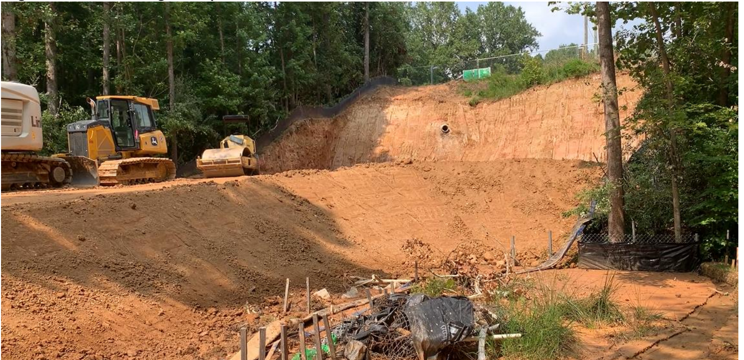
August 7, 2025 Earthen ramp needed for excavating equipment access
