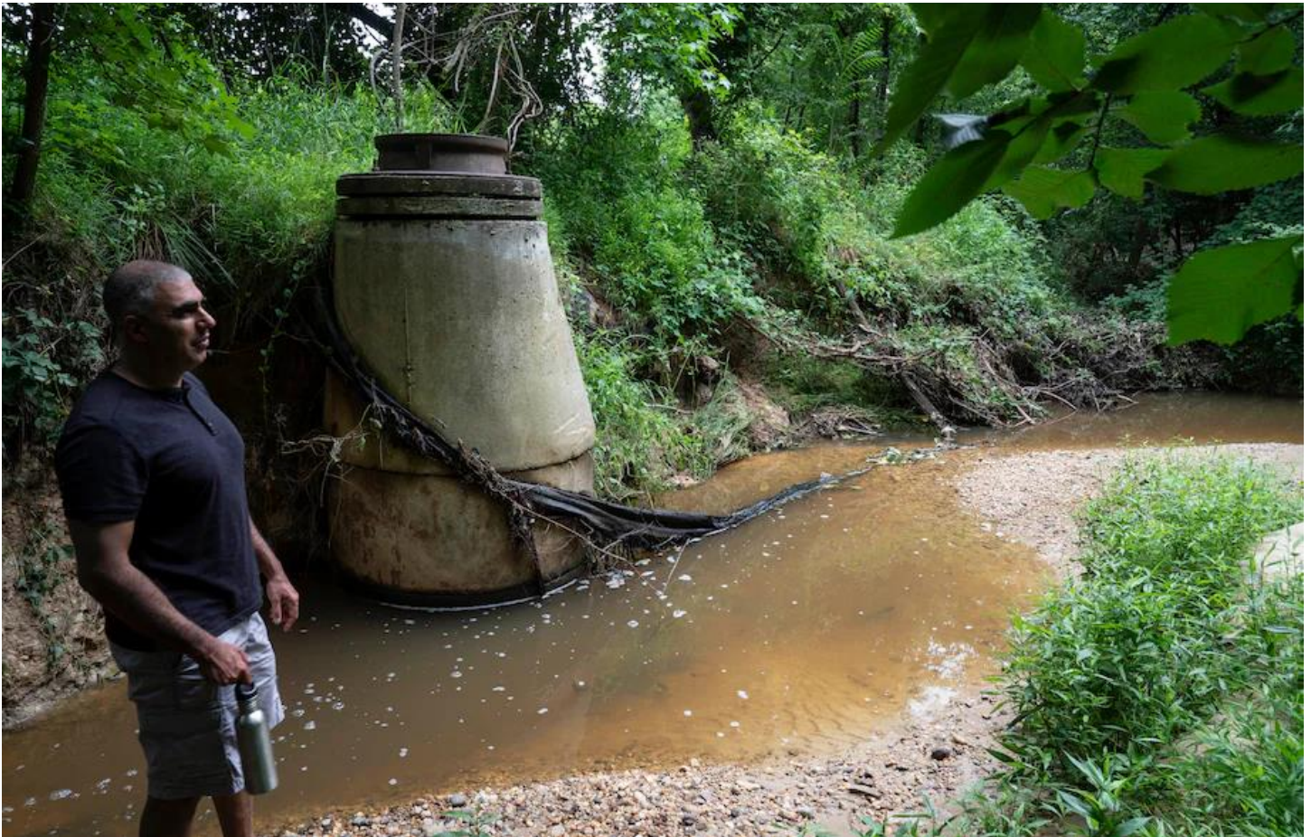
Sujay Kaushal, seen in 2022, stands next to a manhole that has been exposed by erosion along a stream on the University of Maryland's campus in College Park. (Michael Robinson Chavez/The Washington Post)
