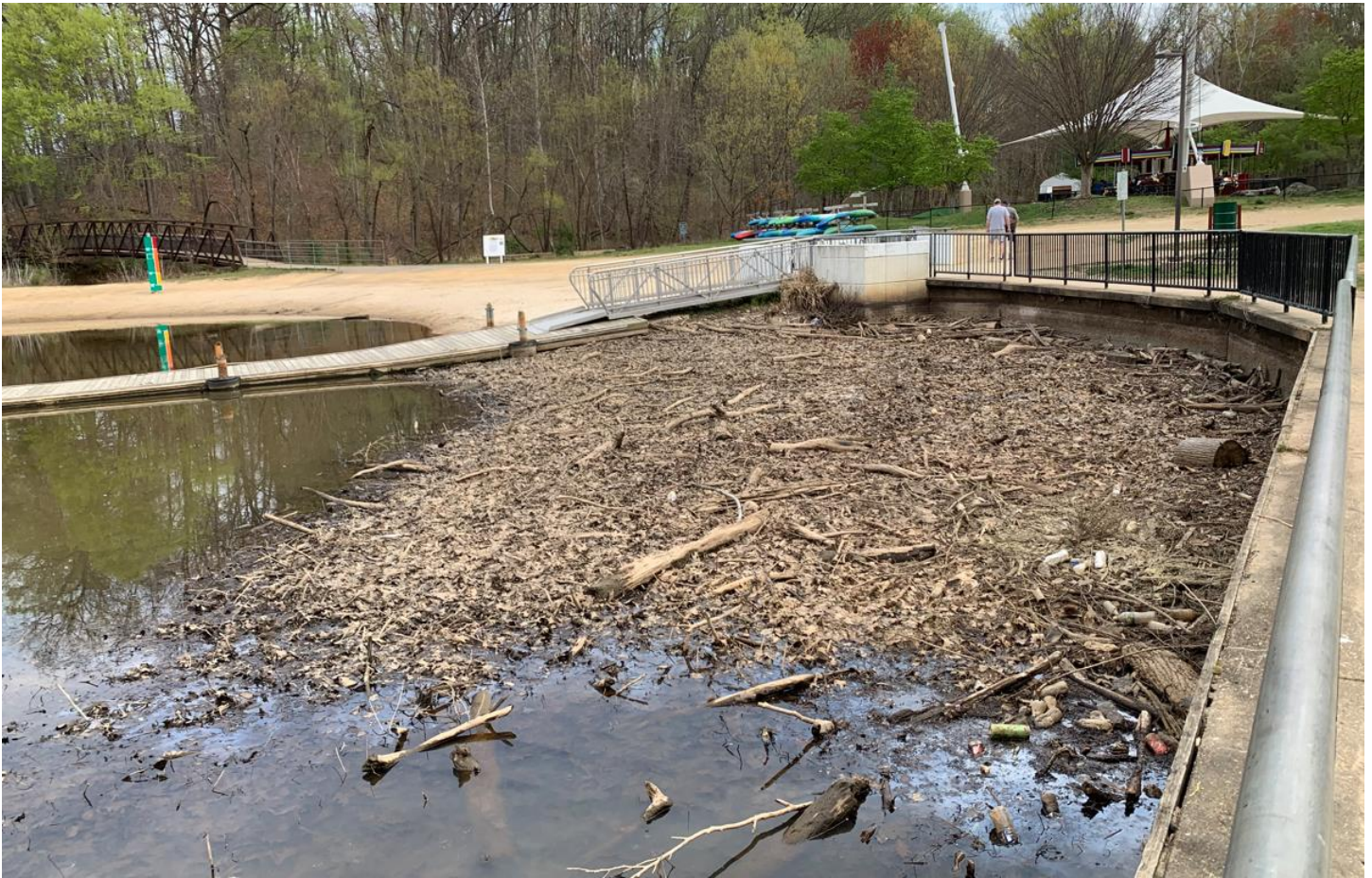
Accumulated organic debris is now above water in the marina
