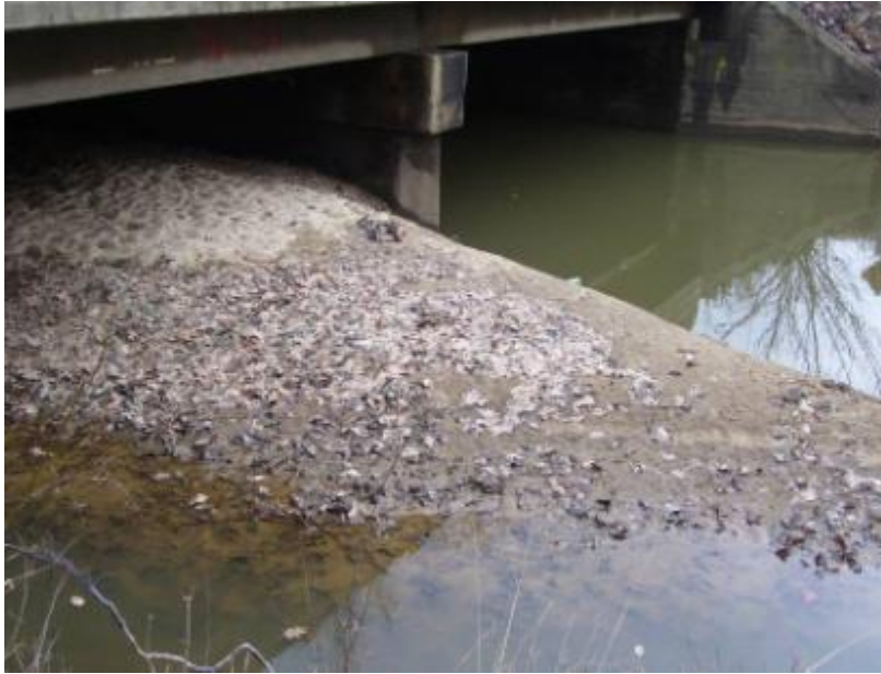
Figure 3-13: Fine Sand Deposit Located Under the Route 1 Bridge over Accotink Creek, near the Tidal/Non-Tidal boundary
