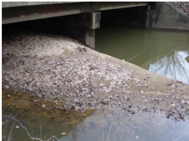
Figure C-2: Fine Sand Deposit Located Under the Route 1 Bridge over Accotink Creek, near the Tidal/Non-Tidal Boundary
