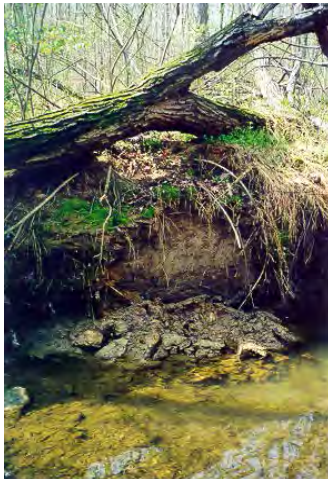
Streambank erosion was common at many locations in the Difficult Run watershed.
