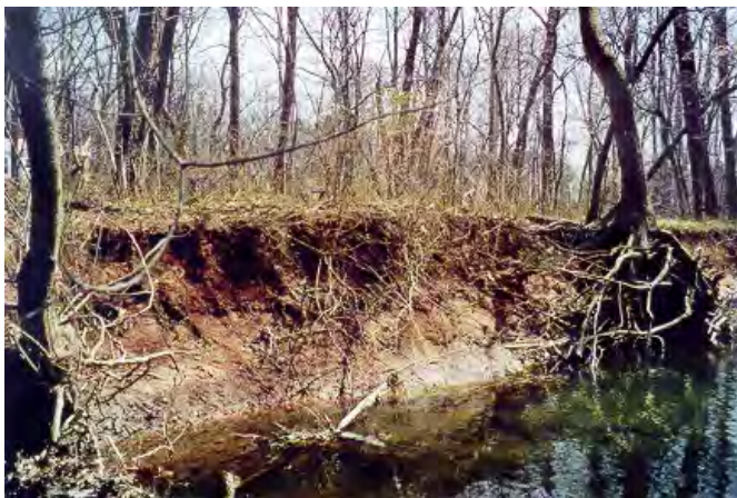
Eroded stream bank and undercut tree root systems are common along the Sugarland Run mainstem.
