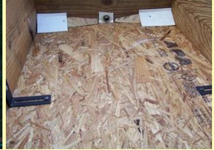
Photo 6 Drain opening and reinforcements
